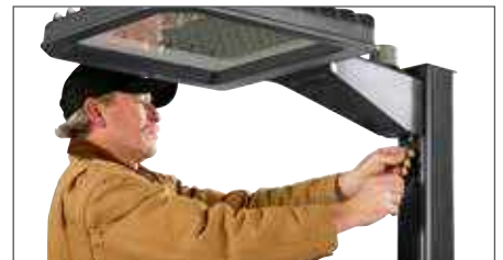
Tighten bottom bolts and complete wiring.
