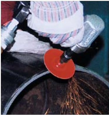
Chamfering the edge of a steel pipe.
