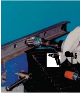
Deburring edges of holes drilled in a C-channel.
