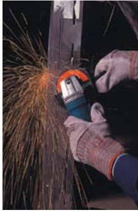
Weld blending after a repair on a steel rack.
