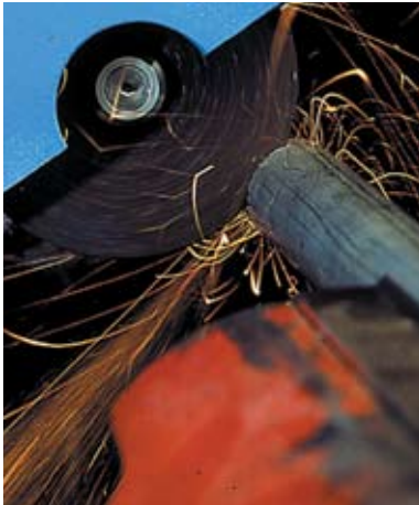
Cutting a length of steel pipe.
