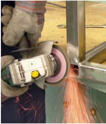
Grinding welds on a fabricated steel part.
