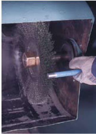
Removing paint prior to welding.
