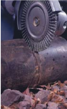
Removing weld slag before the next weld pass.
