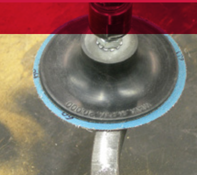
Blending surface imperfections prior to painting.
