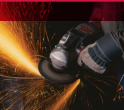
Grinding out weld defects for repair.
