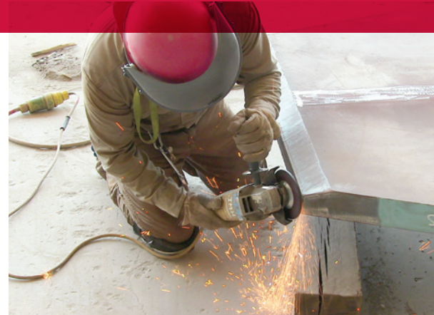
Grinding on a platform for weld preparation.
