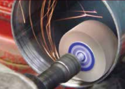
Removing burrs from the inside diameter of a cut tube.
