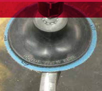
Blending surface imperfections prior to painting.
