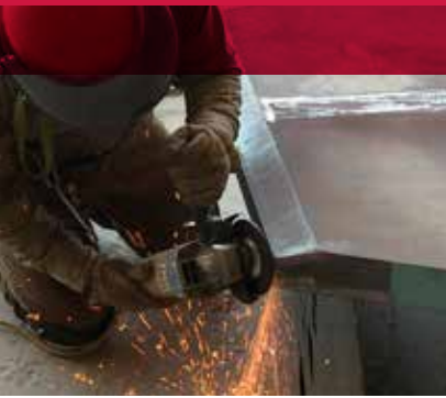
Grinding on a platform for weld preparation.
