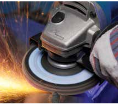
Blending and finishing a weld.
