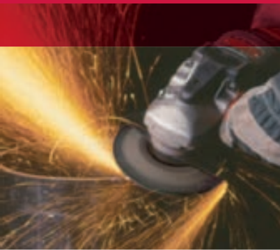
Grinding out weld defects for repair.
