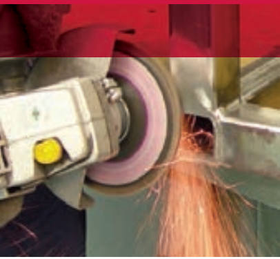
Grinding welds on a fabricated Steel part.
