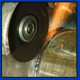
Cutting out weld defects for repair.
