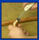
Cleaning the inside of a copper tube fitting prior to soldering.
