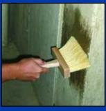
Applying waterproofing material with a masonry brush.
