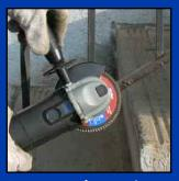
Removing rust from a railing before painting.
