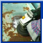
Removing paint & rust from a metal surface prior to painting.
