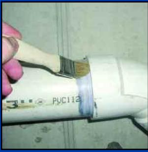
Applying adhesive to PVC plumbing.
