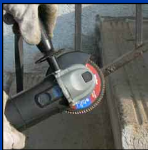
Removing rust from a railing before painting.
