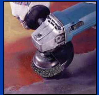
Removing paint from a steel surface with a crimped wire cup brush.
