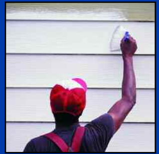
Applying paint to clap board siding.
