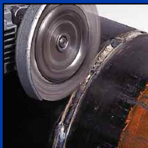
Cleaning a weld with a knot wire wheel brush.
