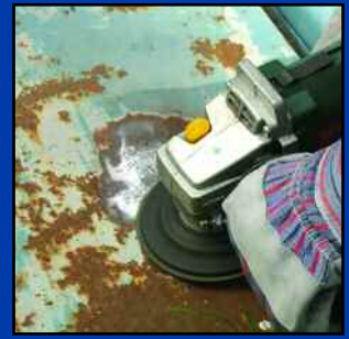
Removing paint & rust from a metal surface prior to painting.
