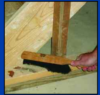
Sweeping dirt and debris from between studs.
