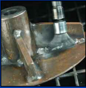
Cleaning hard-to-reach fillet welds on a gusseted base plate.
