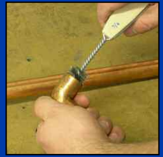
Cleaning the inside of a copper tube fitting prior to soldering.
