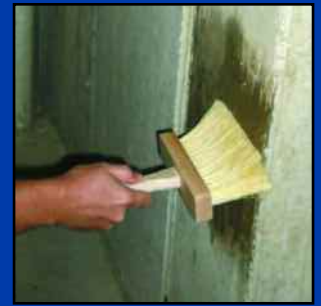
Applying waterproofing material with a masonry brush.
