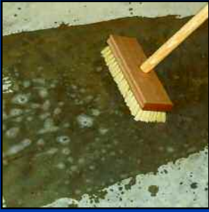
Scrubbing a concrete floor prior to painting.
