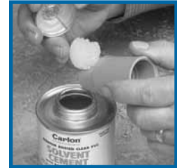
Apply a uniform coat of cement.
