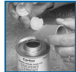
Apply a uniform coat of cement.
