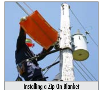
Installing a Zip-On Blanket
