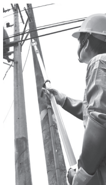
Fig. 3: Voltage detection for overhead lines
