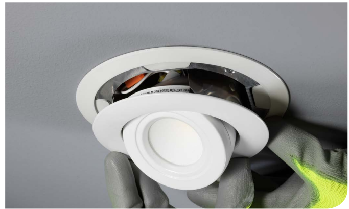
Insert the trim into the housing using push in friction springs and turn power on to the fixture.
