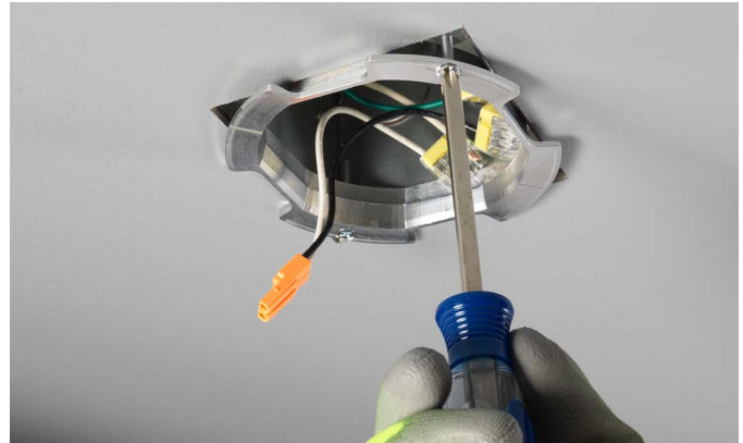
Make electrical connections using stripped supply wires with quick connectors or cap with wire nuts (LED source dependent). Then, secure the mounting bracket to the junction box using the flat head screws provided.
