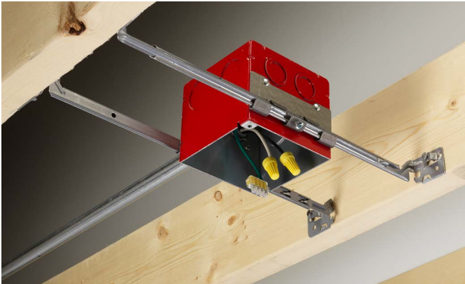
Extend the bar hangers to fit between the ceiling joist and remove the appropriate knock-out(s).
