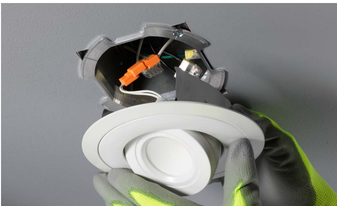
Place provided trim ring around LED retrofit trim and plug the connector provided on the LED trim into the mating connector in the junction box housing.
