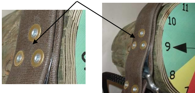
Triangular Rivet Pattern Fig. 3a
