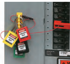
4. For group lockouts, run key through multiple loops in lock rail and apply locks. No hasps required! (Not recommended for use with multilock hasps)
