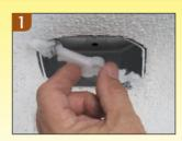
Back the screws out enough to slip the bracket on.
