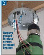
Drill (2) 1/8" diameter holes into joist through the elongated openings on each side of box. Remove the (2) long screws noted above to mount the fan/fixture bracket.
