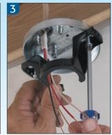
Mount the fan/fixture bracket into the drilled holes. And you're ready to install the fan or fixture.
