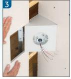
Cut and position drywall to fit around the box. (Note: captive screws in box.) Install fan or fixture per manufacturer's instructions using captive installation screws.
