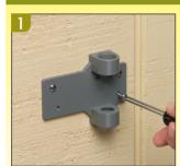
Mount conduit adapter plate in desired location using three screws (not provided)
