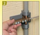
Insert grounding electrode conductor into the lay in lug. Tighten screw.
