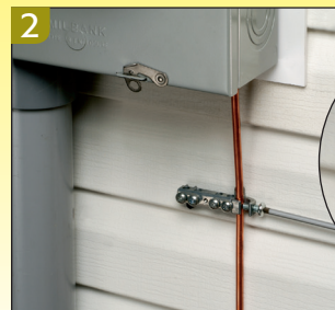
2 Insert grounding electrode conductor into the lay in lug. Tighten screw.
